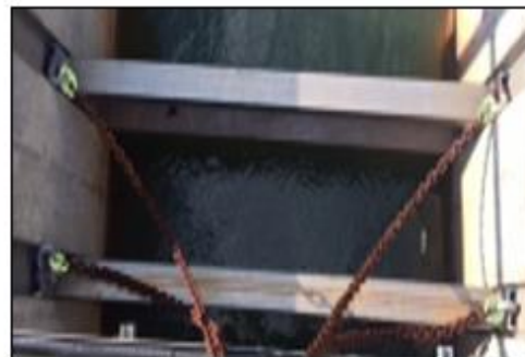
Embedded in Concrete
