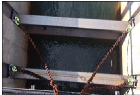
Embedded in Concrete
